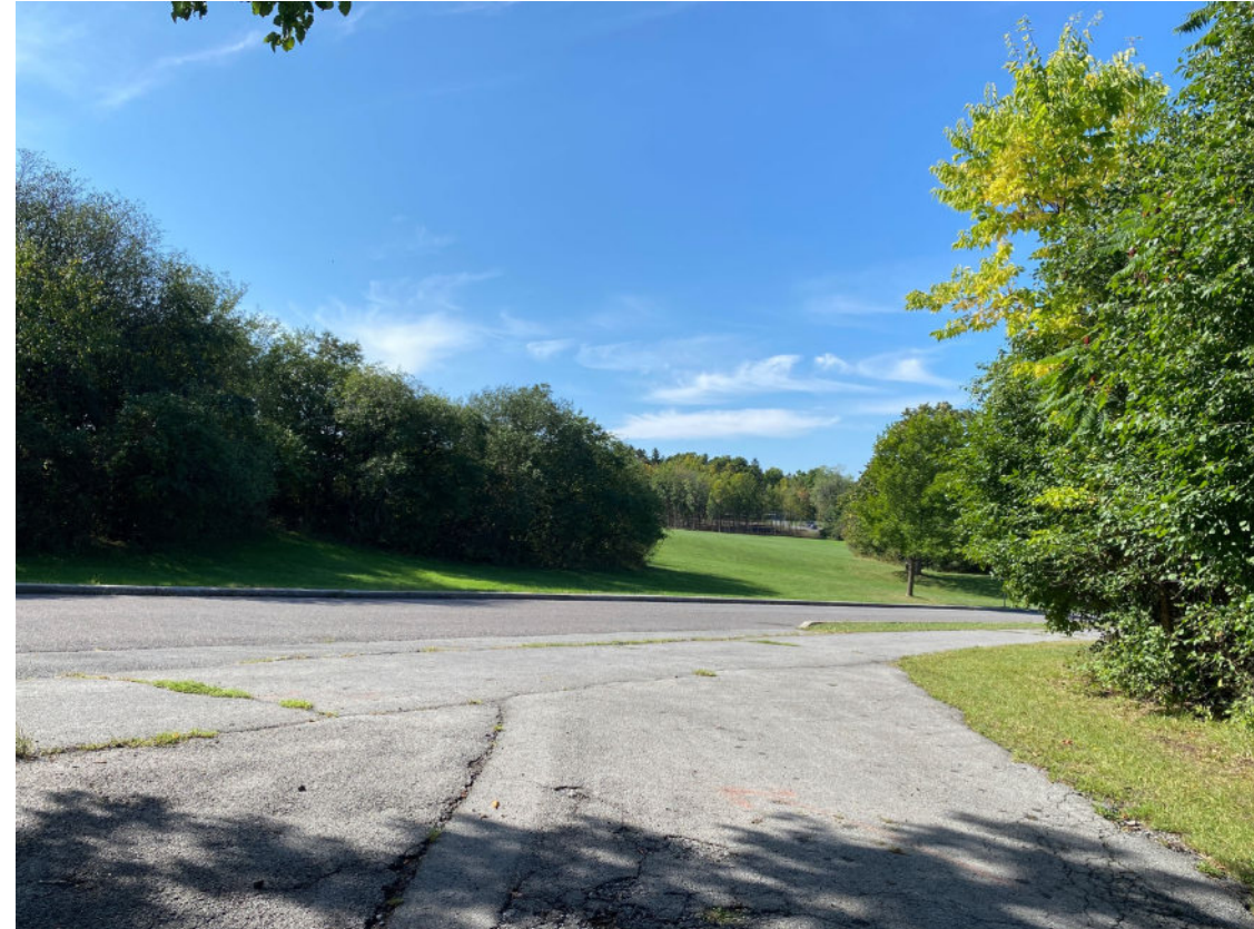
Intersection of pedestrian path and roadway with excess pavement.
