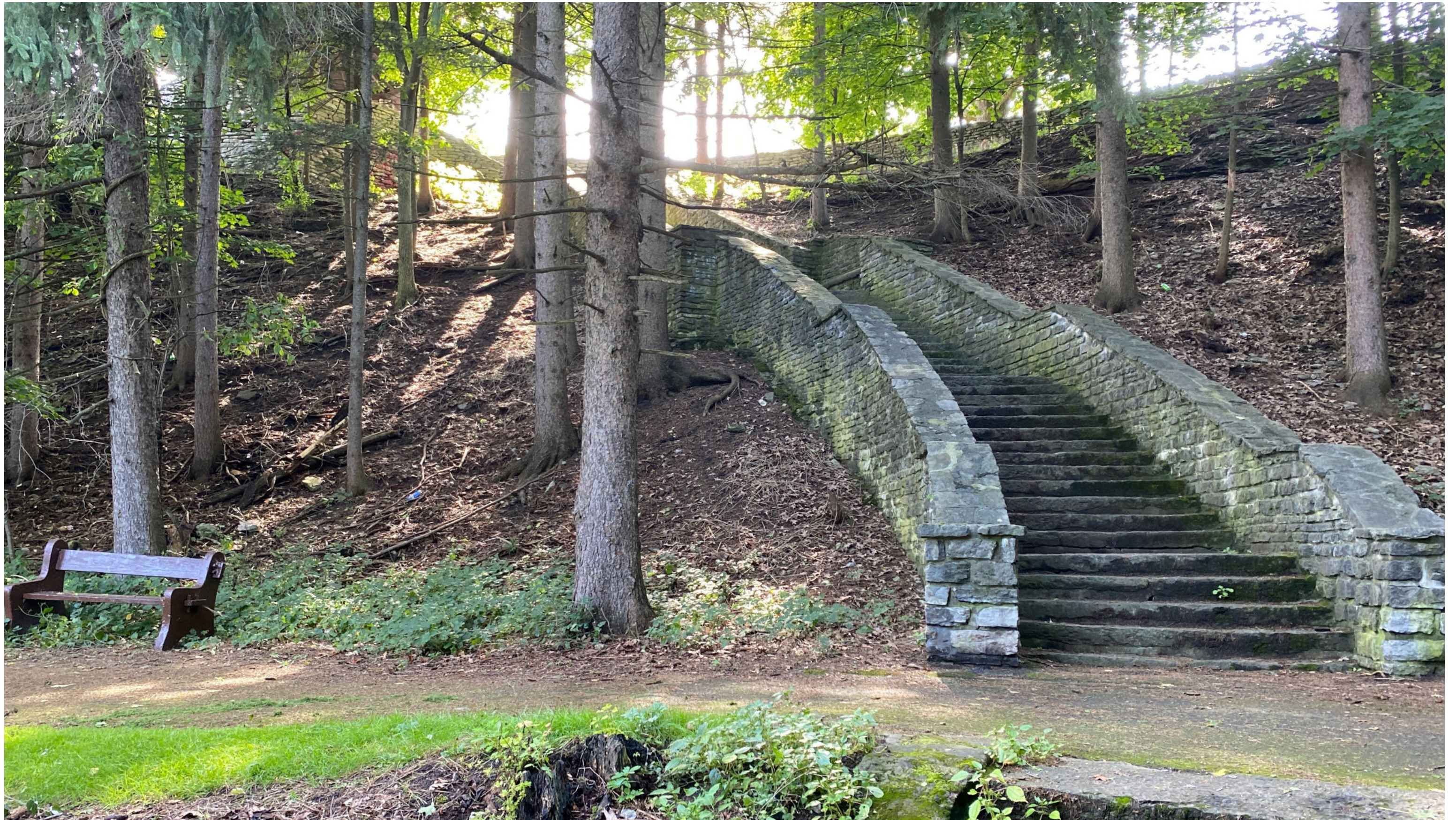
View of the existing historic stairs which lead to the core of the park, also known as the Olmsted Acres.
