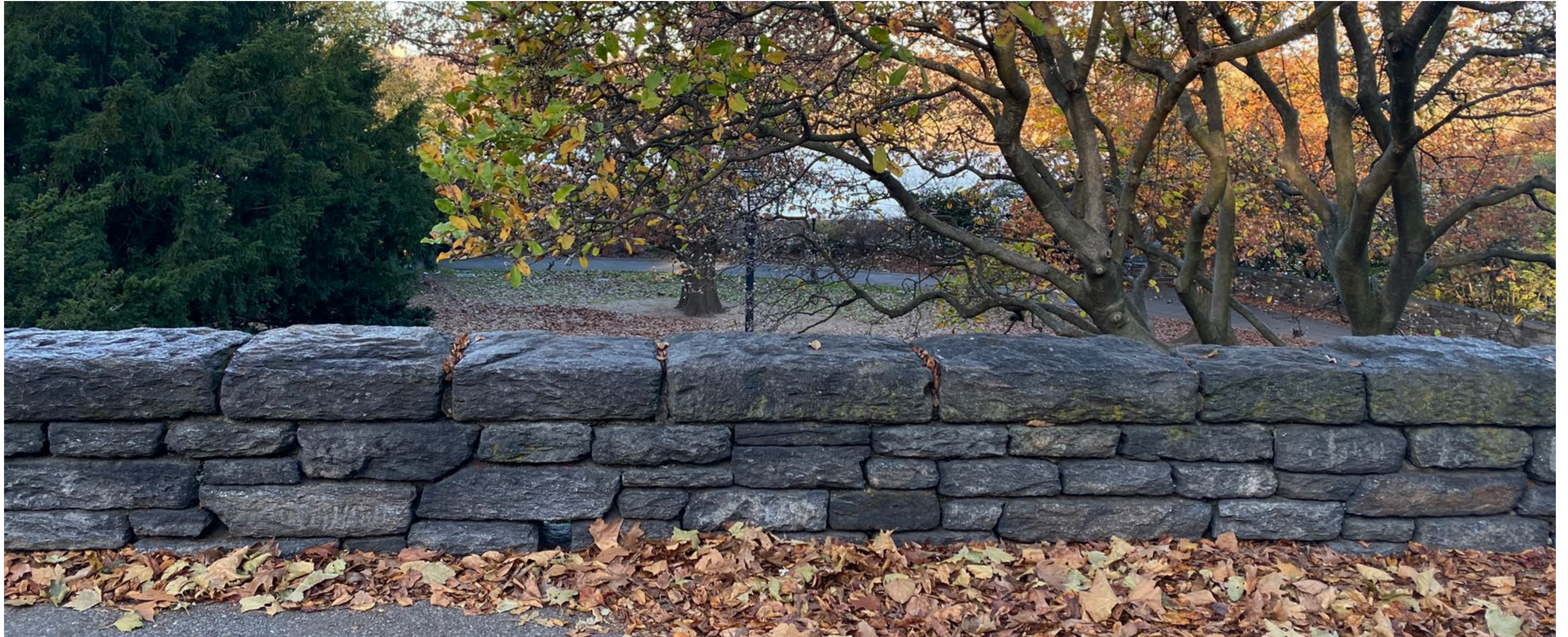
Frame edges and entrances with low masonry walls and piers.
