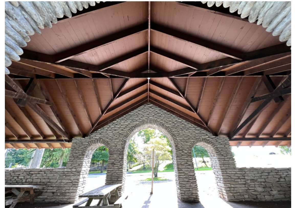
11 Interior view of Picnic Pavilion
