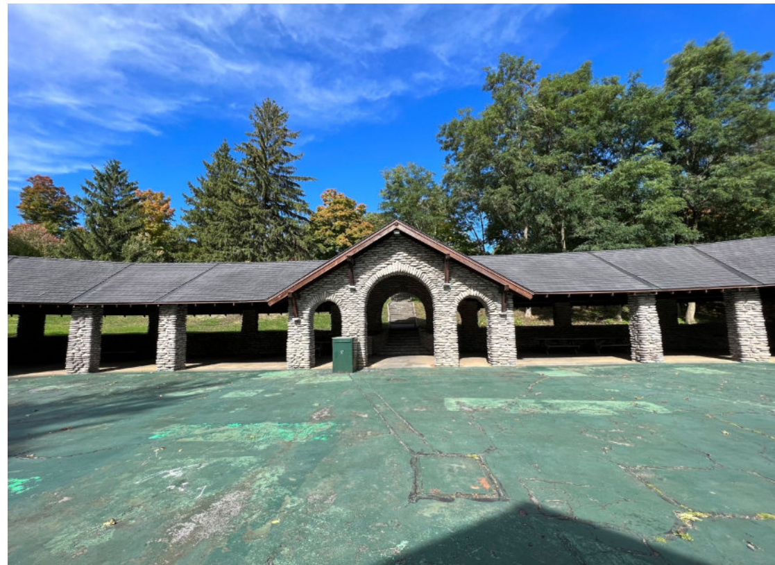
11 Interior pavement and event access to Picnic Pavilion need improvement.
