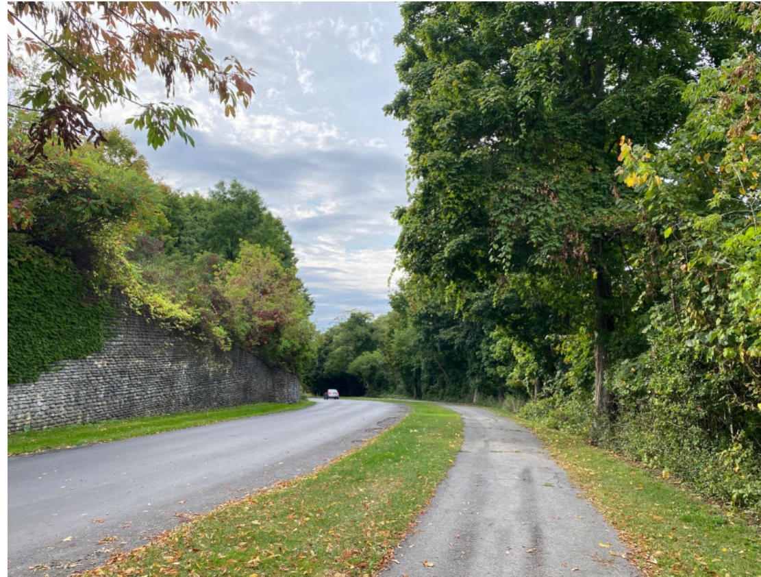
Paved path system which runs parallel to the loop drive
