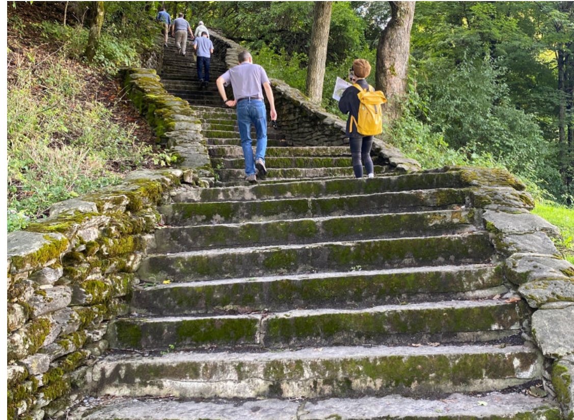
1 Existing stone stairs with monolithic stone treads.
