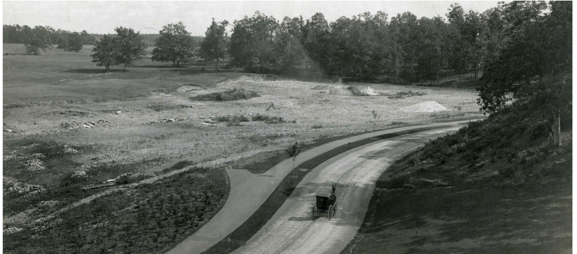
Park paths and drive under construction, 1902. Image Courtesy of the NPS, Frederick Law Olmsted National Historic Site
