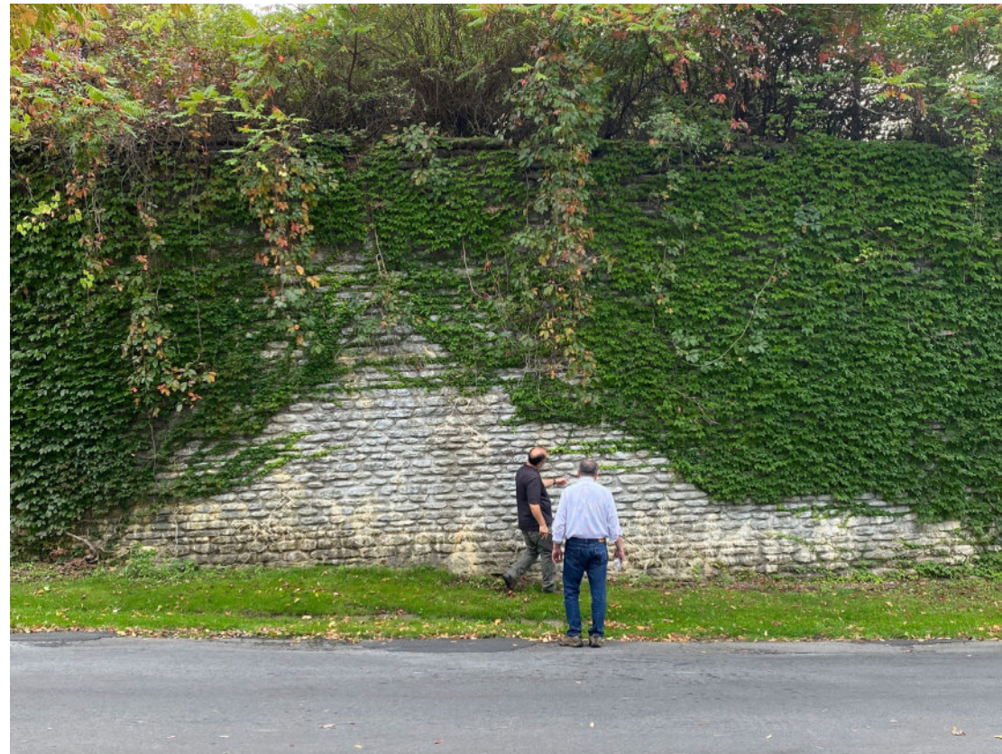
3 Existing retaining wall lighter portions exhibit calcium efflorescence
