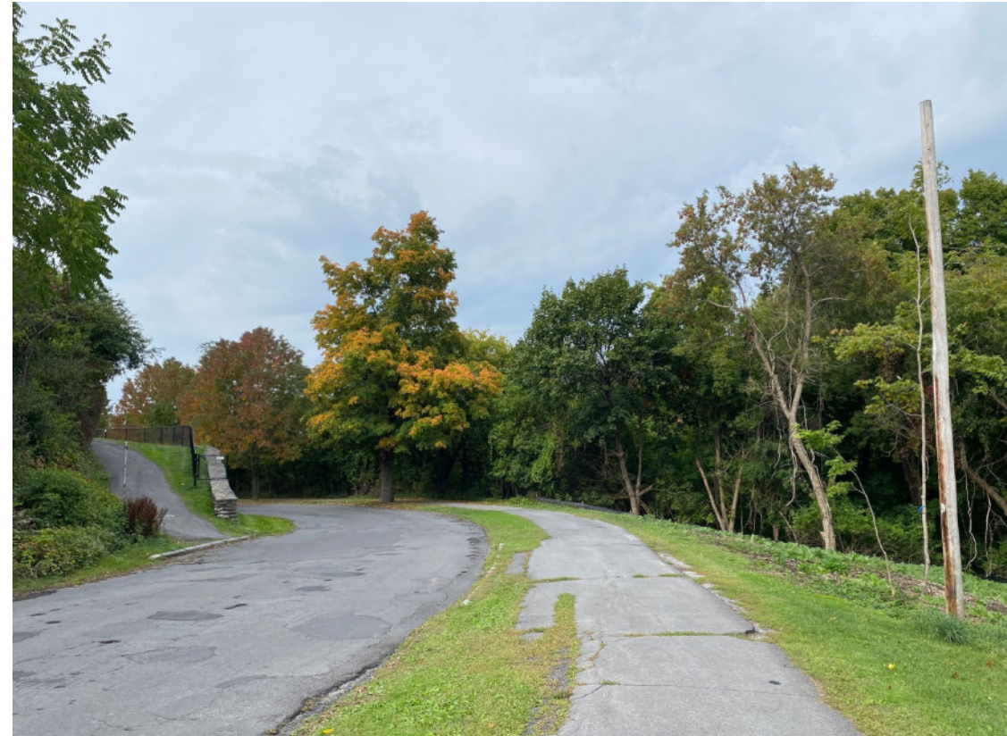
Parallel Roadway and pedestrian/bike path, margins showing multiple layers.
