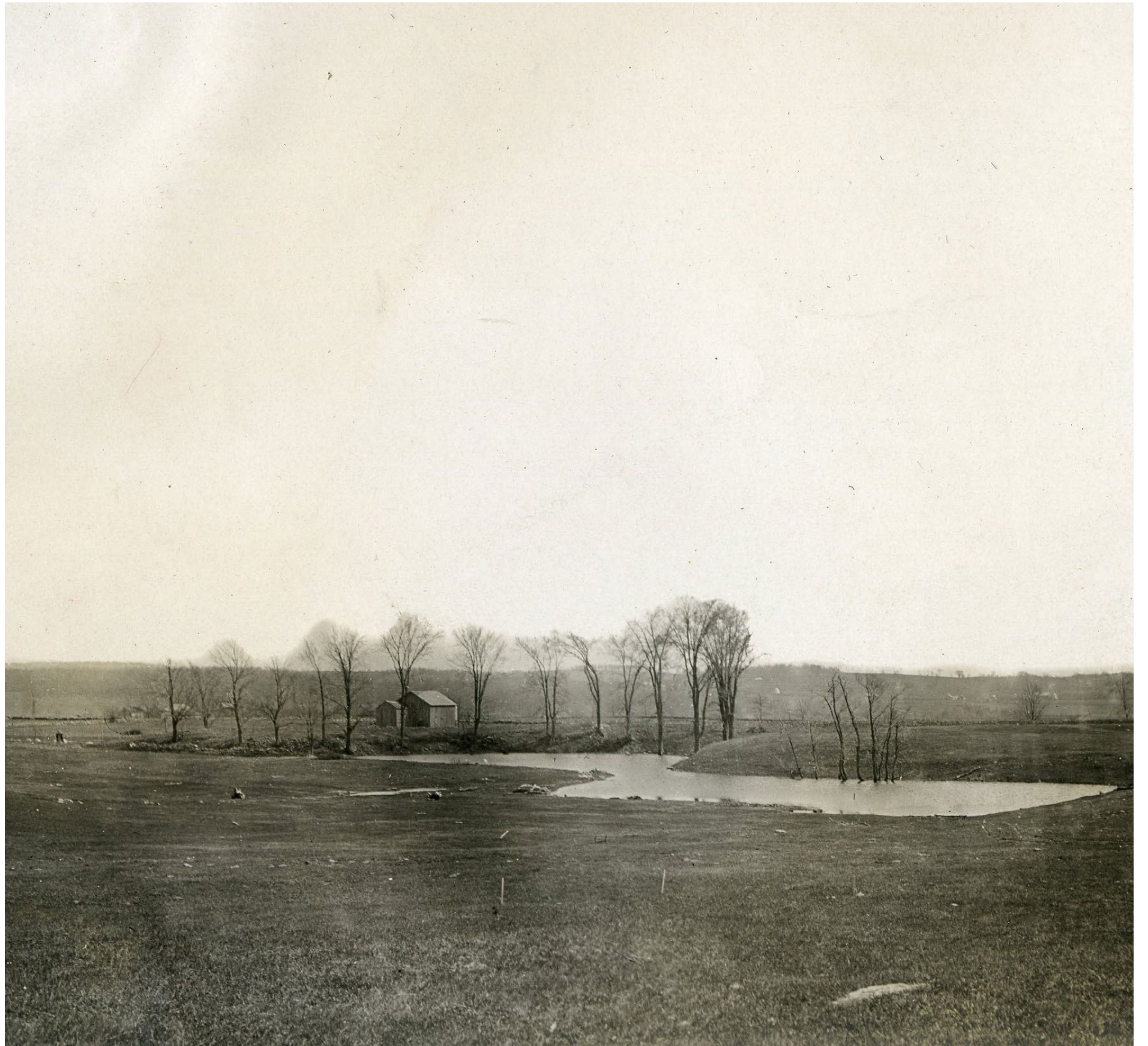
Ephemeral waterbody on the farmland pre-park construction, 1899. Image Courtesy of the NPS, FLO National Historic Site
