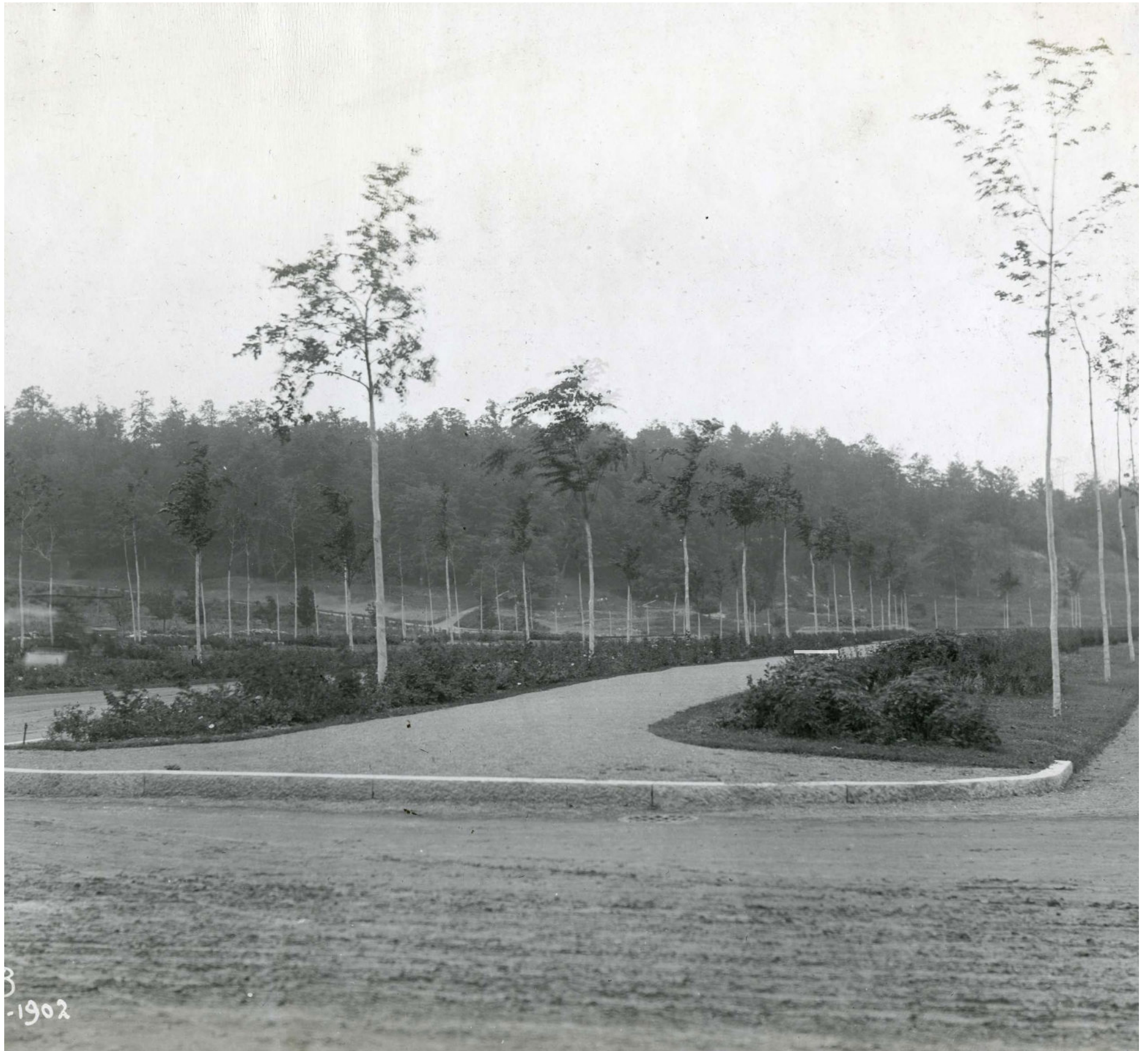
View of tree allee on Academy Circle, shortly after installation, 1902
