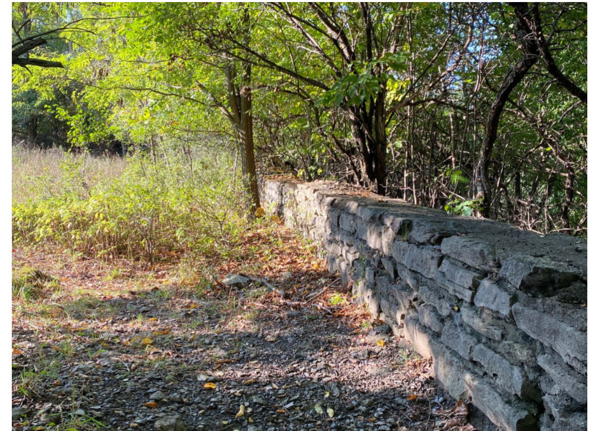
4 Existing masonry retaining walls could benefit from stone caps.
