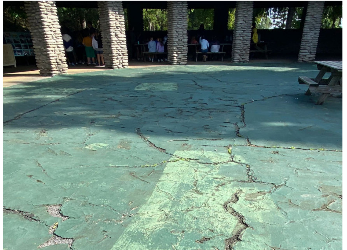
Pavement within the Picnic Pavilion
