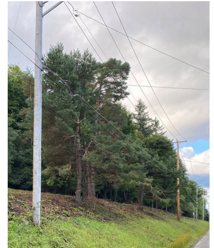
+ Street Lights - Wooden Pole
