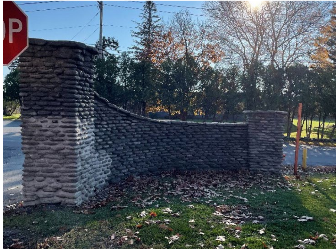
1 Grout not consistently colored on masonry walls
