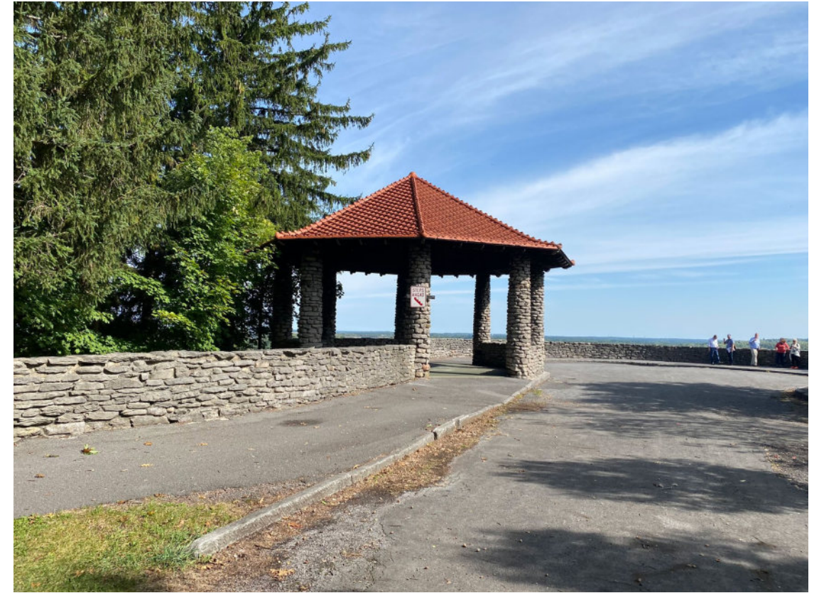
9 Pinnacle Overlook road pavement and curb need alignment.
