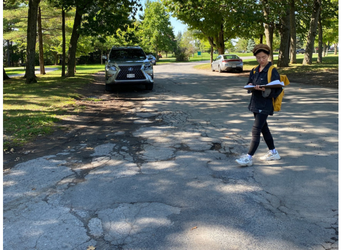
Edge of road degraded by off road parking
