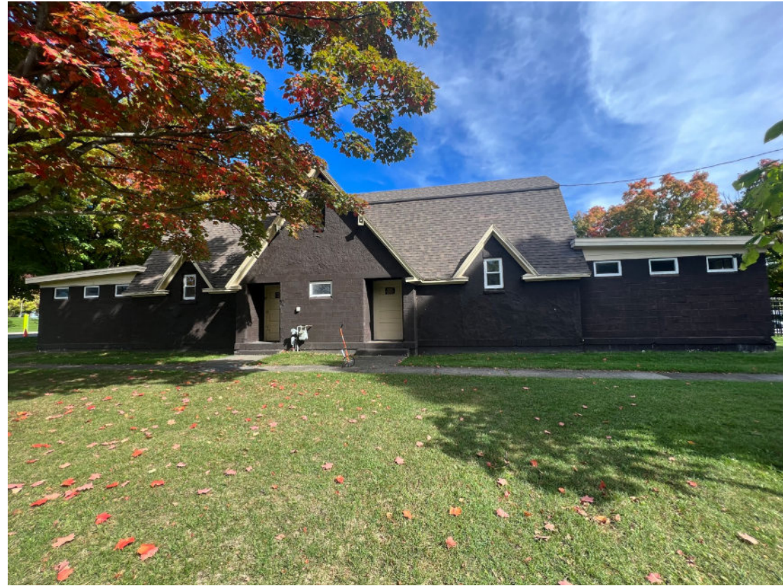
15 Old Bath House - currently closed and in need of rehabilitation.
